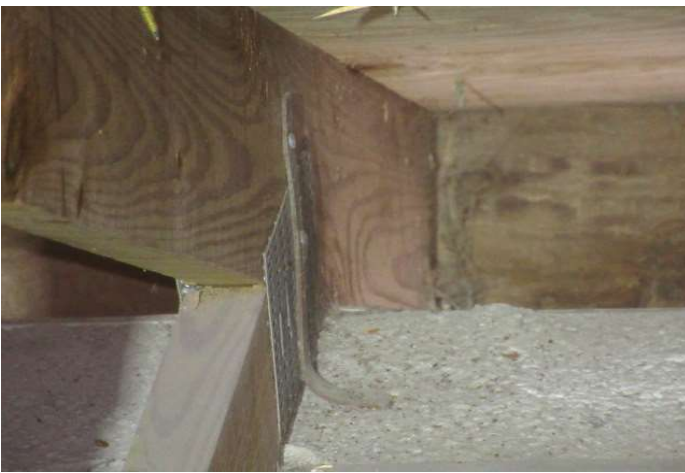
Single strap with 2 nails into the truss
