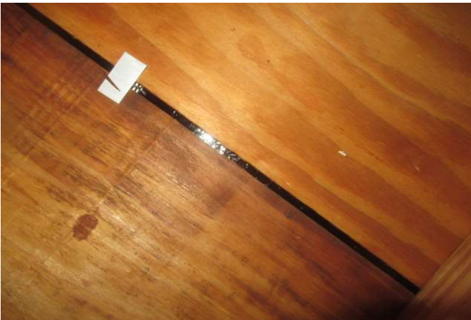
SWR installed under the tile
