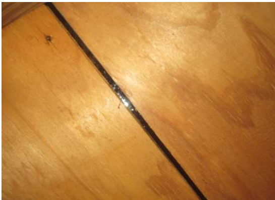
SWR installed under the tile
