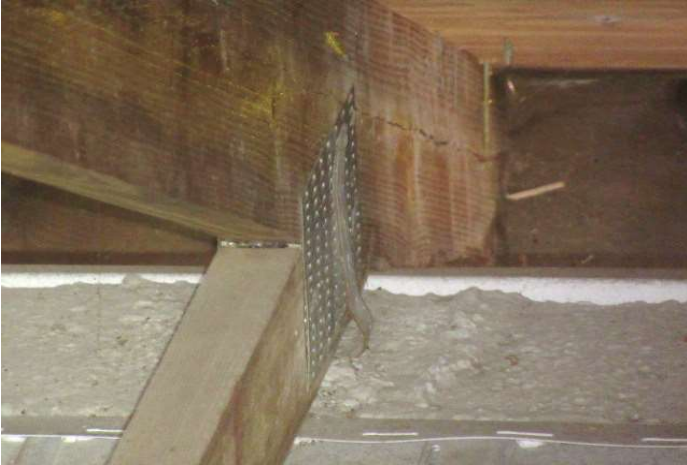
Single strap with at least 3 nails into and through the truss
