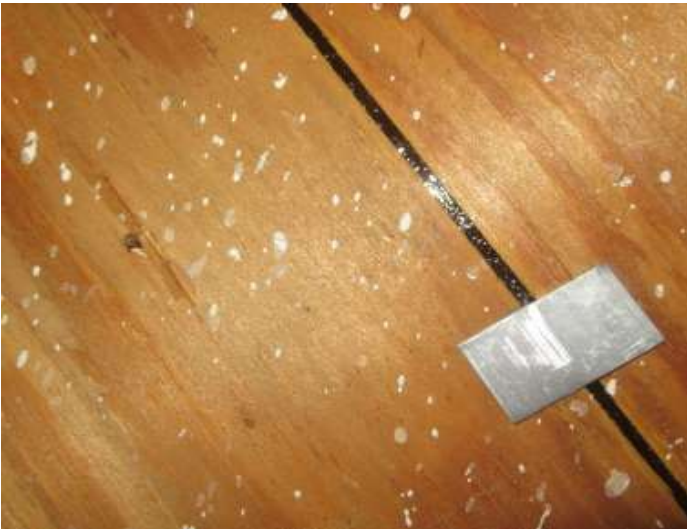
SWR installed under the tile
