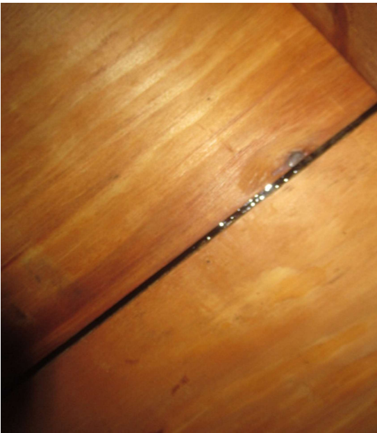
SWR installed under the tile
