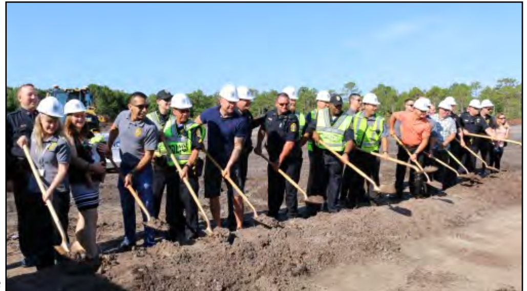
Members of the Venice Police Department turn a ceremonial shovelful of dirt at the May 17 groundbreaking ceremony for the new Public Safety Facility.
